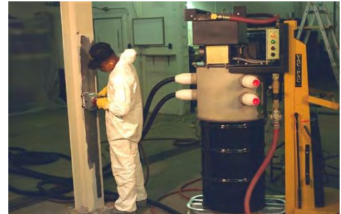
Worker is using the roto-peen (scabbling) attachment; VAC-PAC collection system shown with 55 gal drum.
