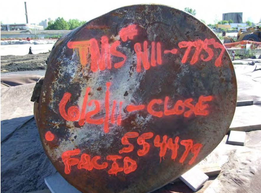
Photo 8 – View of end of 2,000-gallon UST. Note, UST was cut-up on-site at a later date and bulked for disposal with other metal debris excavated during IRM #1 activities.
