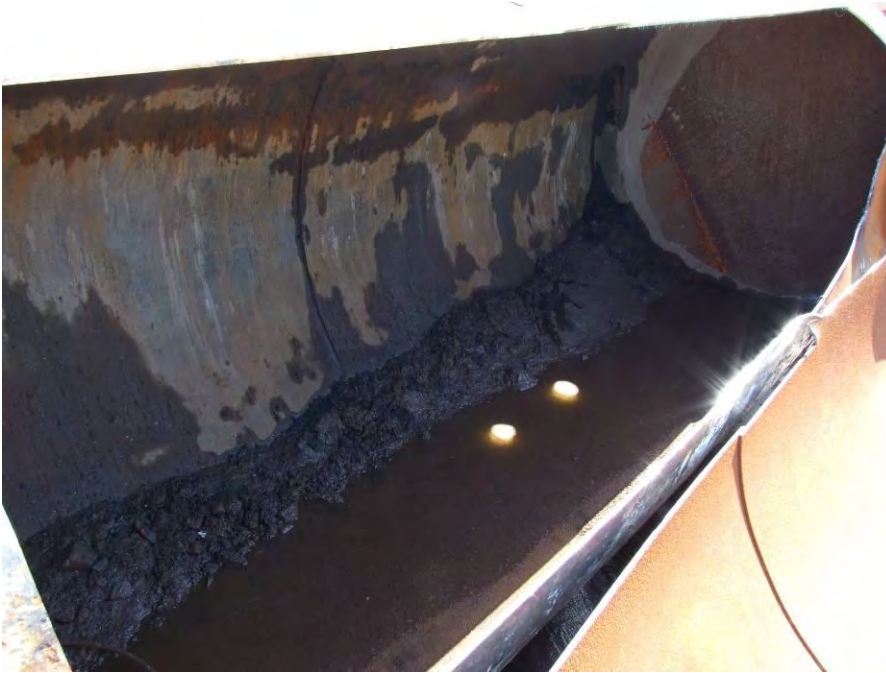
Photo 15 – View of sludge and liquid remaining within the interior of the 1,000-gallon UST. Note, two port holes were open when the UST was discovered.
