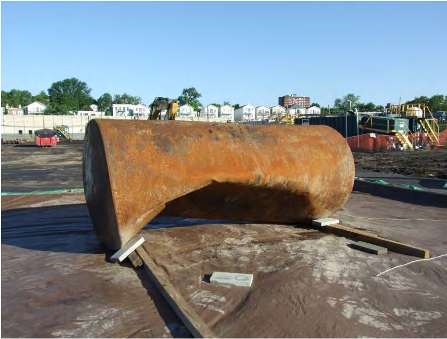
Photo 1 – View of 2,000-gallon UST removed from IRM #1 Grid B1B.
