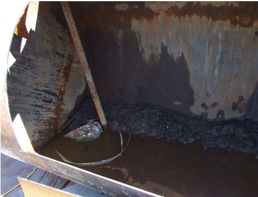
Photo 14 – View of sludge and liquid remaining within the interior of the 1,000-gallon UST.
