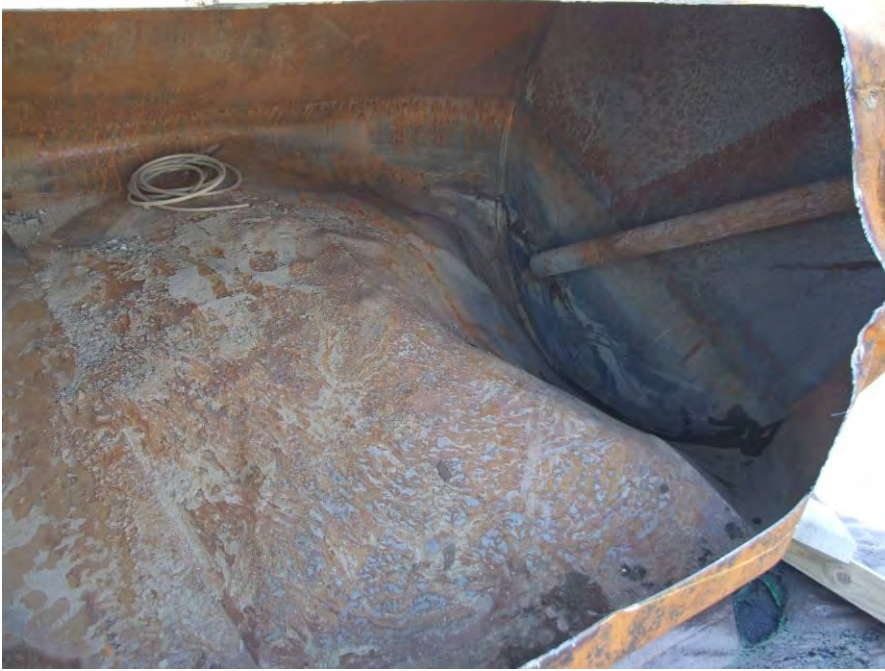
Photo 6 – View of 2,000-gallon UST interior after cleaning (opposite end from Photo 5).
